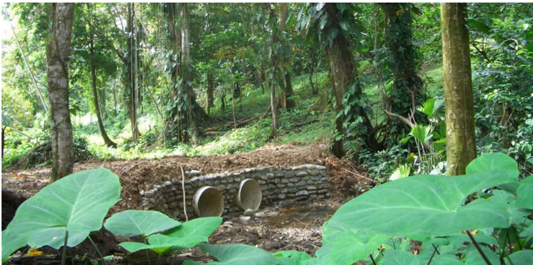
4mar06 - Rough Grade almost complete, only landscaping remains.
