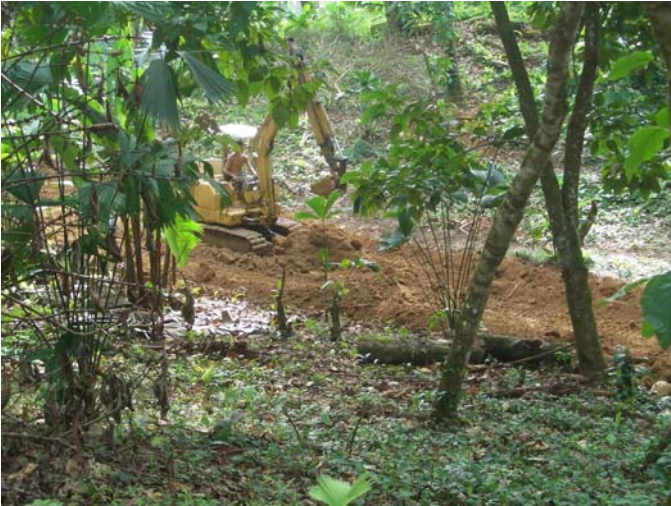
26jan06 - Excavator works well for this type of work.
