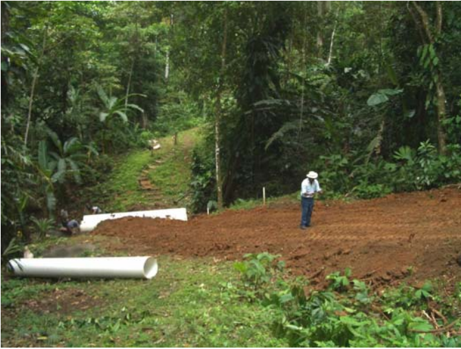
7jan06 - Looking West on Via Monte lots 3-4, Prestan telling operator where to add fill
