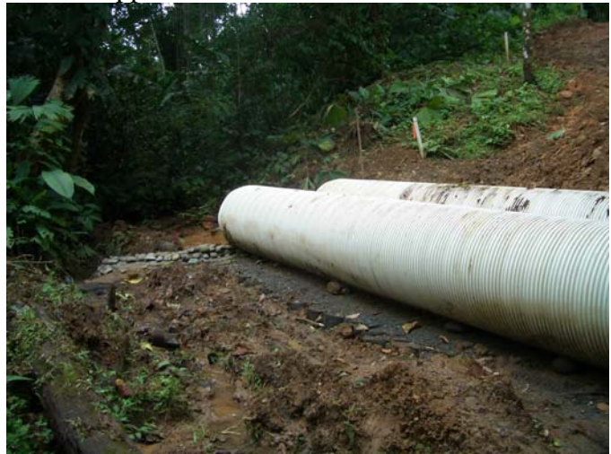
17jan06 – Culvert on GeoWeb Pillow and diversionary ditch at bottom center left
