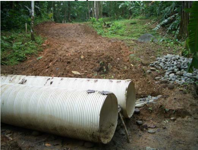
17jan06 - looking East from culvert base, Head wall footers are in place, road base will be 1m above culvert eliminating ravine
