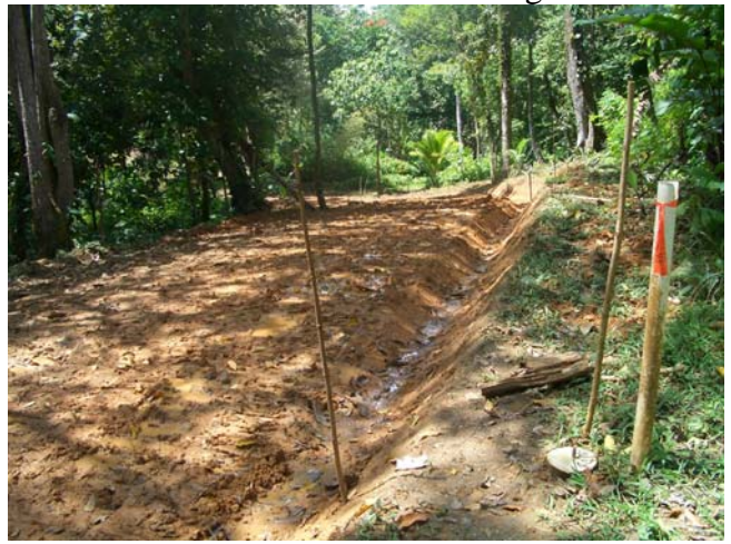
25feb06 – looking west from lot 44-45, the ditch takes lot run off water to a culvert near lot 46
