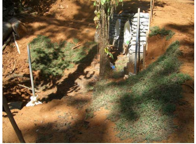
10feb06 – looking west on Via Monte at Culvert Bridge at lots 1-2
