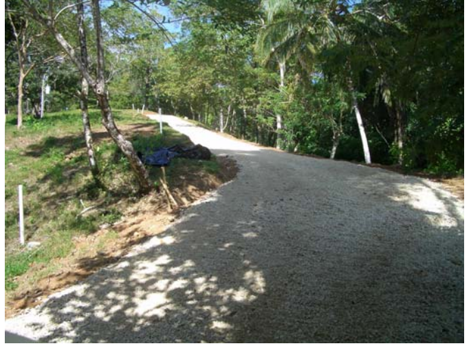
Cart Path base aggregate at Lots SB32, SB41, SB42, and SB43
