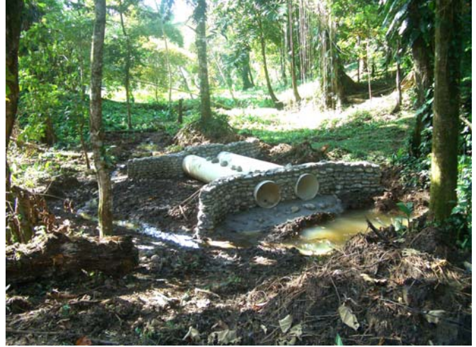
Culvert pipe has been installed and stone headwalls are in place
