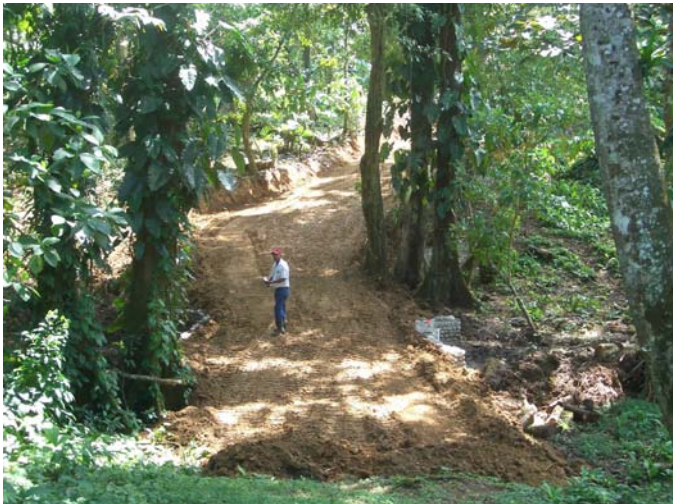
The final Rough Grade over the previous photographed culvert
