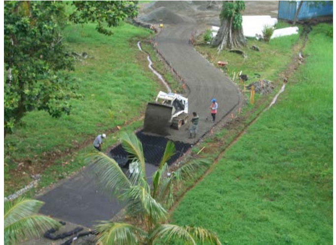
This 91 meter section was completed in a day and half.
